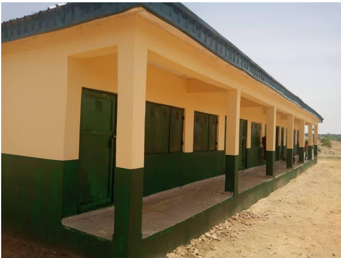
Newly constructed classroom blocks at LGEA Mahuta
